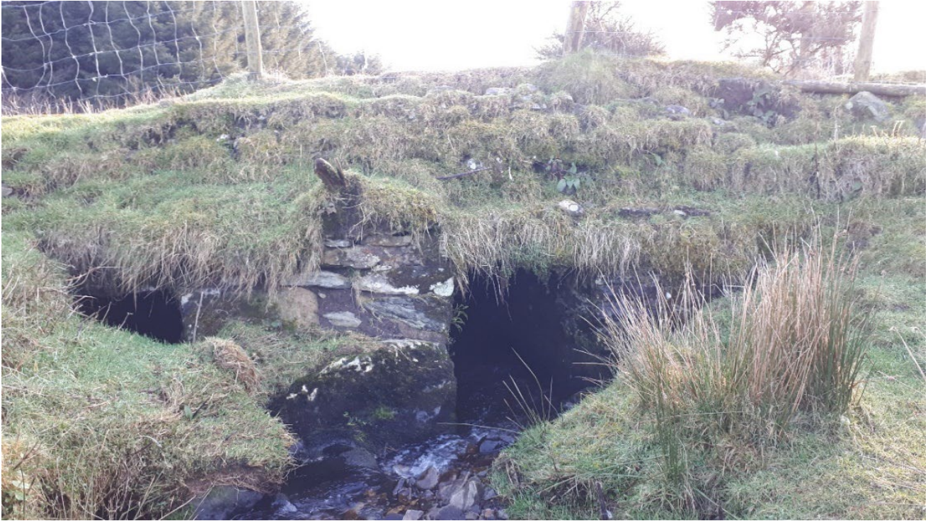
Figure 3-14: Existing Stone Bridge Crossing (WF-HF8)
